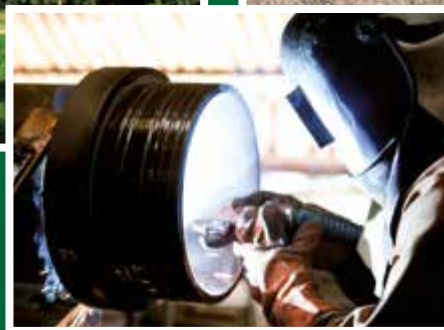
Welding of the spigot end and pipe
