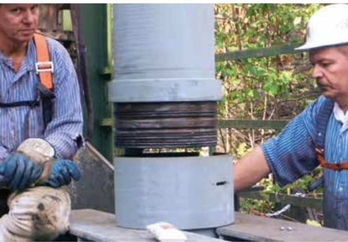
Installation of a ZSM Pipeline
